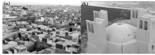
Fig. 5 (a) High density of construction in hot and arid region of Iran, (b) The two-sided wind-catcher and domed roof as reservoir
