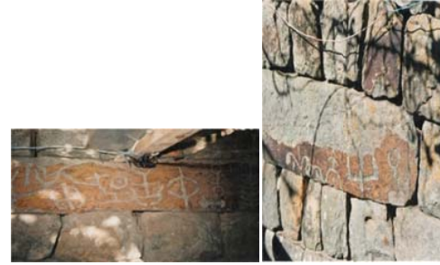
Fig. 4 Masterpieces used in construction
