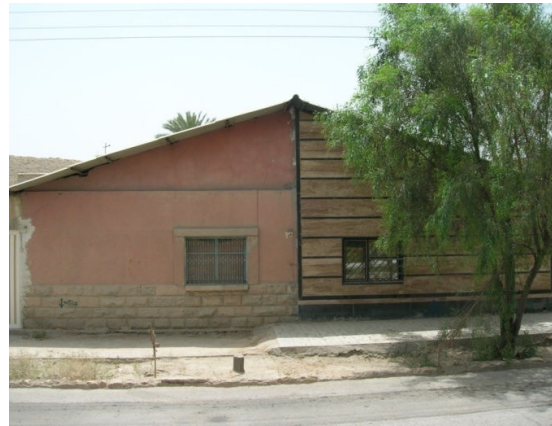
Fig. 8 Twin prefabricated houses in New Lar city
