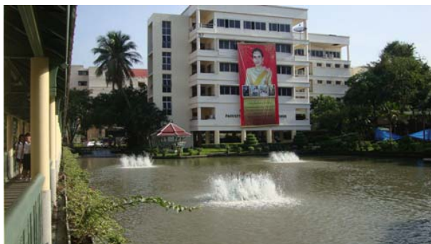
Fig. 1 Operation of Some Surface Aerators in Suan Sunandha Rajabhat University
