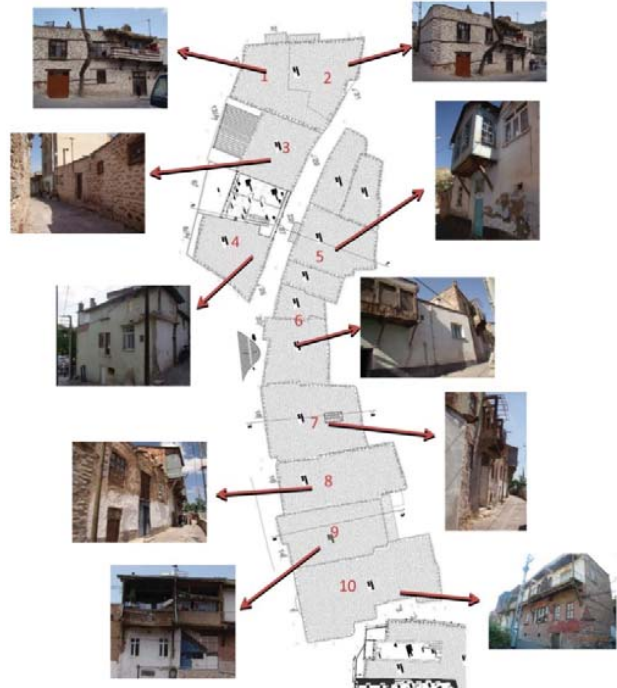
Fig. 3 10 Houses determined as the working area
