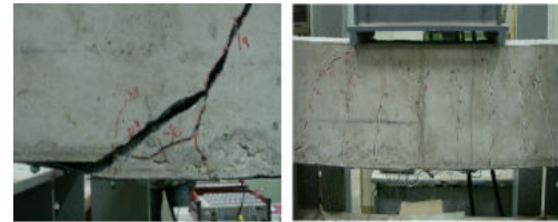
Fig. 14 Anchored aluminum strengthened RC structure failure mode
