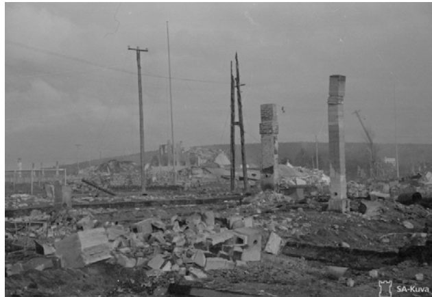
Fig. 2 The destruction of WWII was heavy particularly in Northern Finland. As a result of the war some 40–47% of the dwellings in the area were destroyed, and the provincial capital of Rovaniemi was burned to the ground (SA-Kuva)
