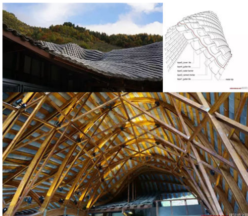
Fig. 8 The roof of volunteers' house of Cattle Hill
