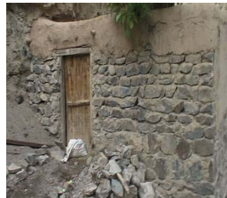
Fig. 6 Stone in the building's walls
