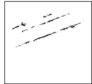
FIGURE 7 ISOLATED CRACK DEFECT TILE IMAGE USING CRACK DEFECT DETECTION ALGORITHM
