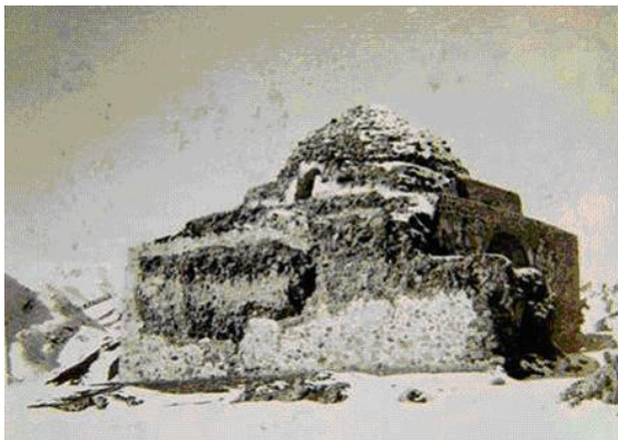
Fig.38 An image of eastern wall of cross-vault "Baze-hur" before mending and the hole created on it
