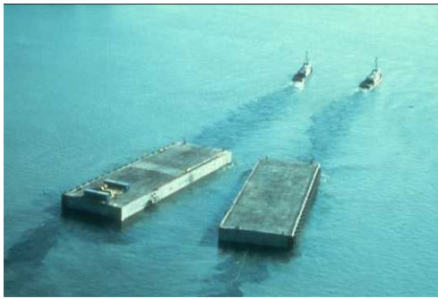
Fig. 3 Towing of pontoon modules [3]
