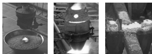
Thermit powder Welding process welding joint
