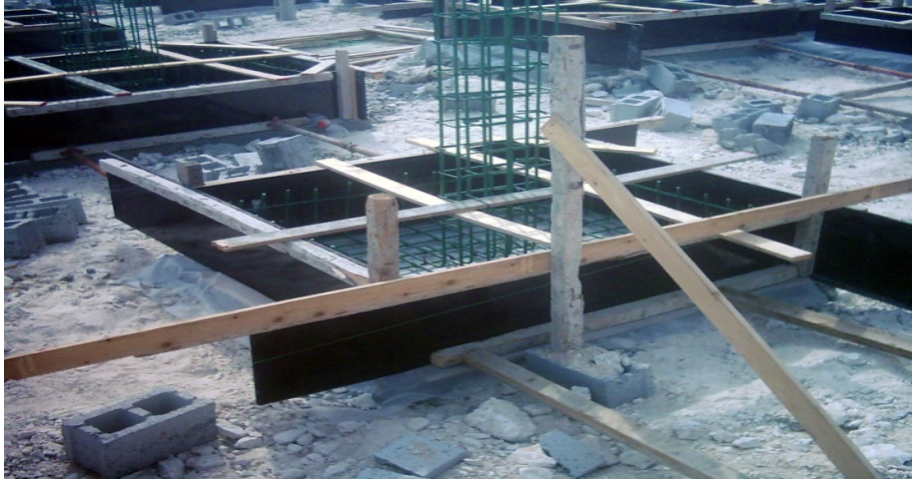
Fig. 4 Footing formwork material – Four sides
