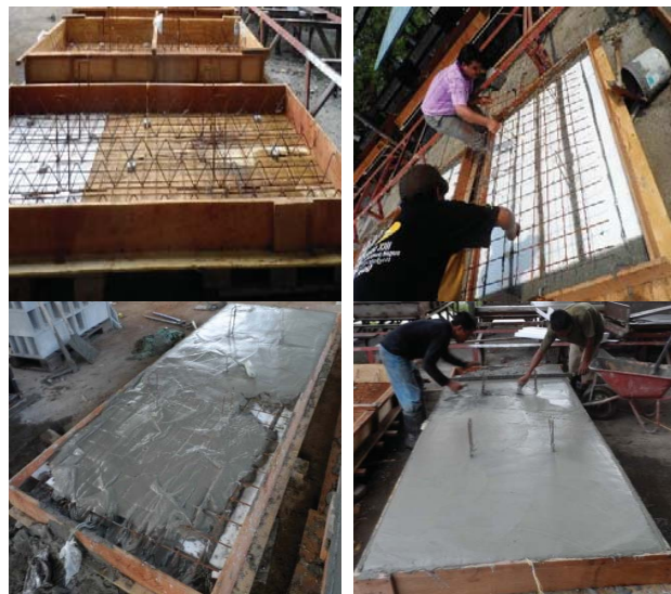
Fig. 3 Preparation, fabrication, and casting of PFCSP specimens
