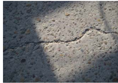
Fig. 10 Deck Damage
