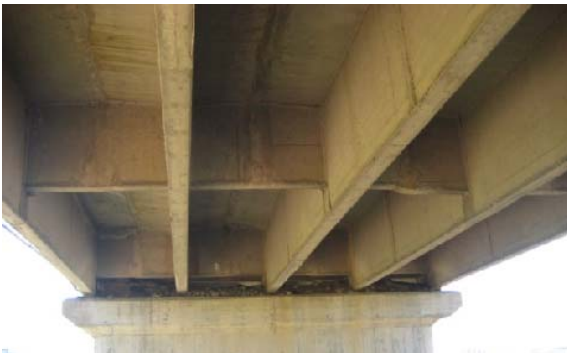
Fig. 9 (d) T Beam connections is good, no obvious damage (diaphragm)
