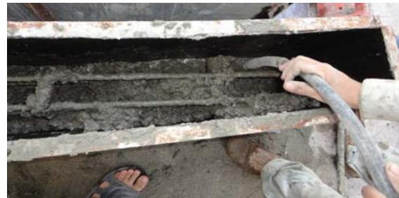
Fig. 4 Compaction of concrete in moulds with vibrator
