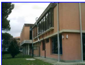
Fig. 10 Views of the building before the seismic retrofit and architectural renovation interventions
