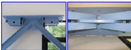
Fig. 19 Final half-stroke positioning of a spring-damper, and views of the same DB panel
