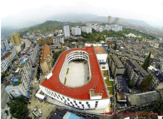
Fig. 1 Roof playground in a primary school
