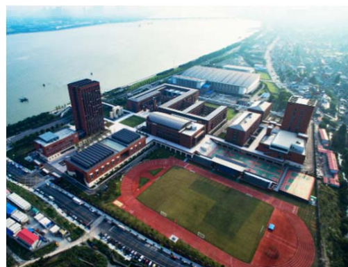
Fig. 4 Site situation of Hangzhou Senior High School Campus
