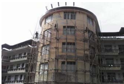
Fig. 2 Reconstruction due to original unreasonable design
