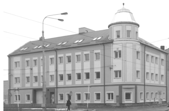
Fig. 1 Technology Centre of Ostrava in Czech Republic
