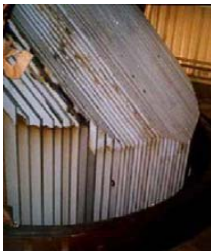
Fig. 4 Case of current circulation in the core
