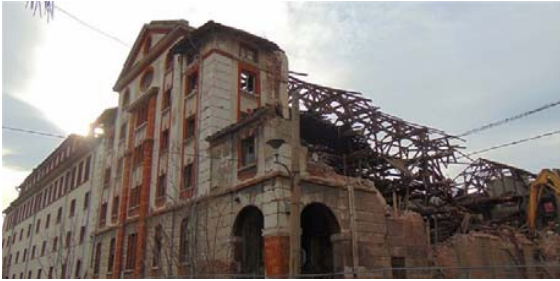
Fig. 7 The partially demolished tobacco warehouse [14]
