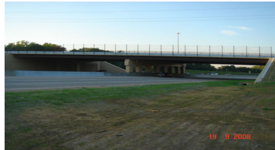
Fig. 1 Pacific Street Bridge, Omaha, NE
