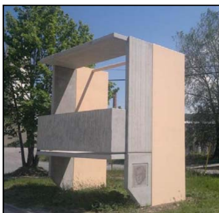
Fig. 4 Real construction of a self-supporting loggia
