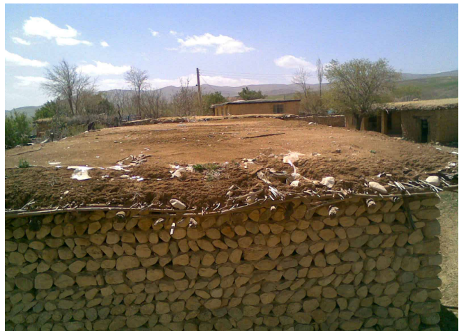
Fig. 4 using the terraced roof and an insulator made of clay and straw (Hamedan, Iran)
