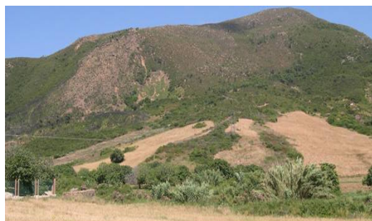
Fig. 5 Landslide interesting pouring - Valley Ksar es Shrir
