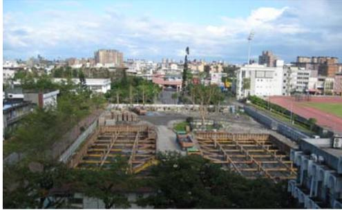
Fig. 2 Excavation construction support
