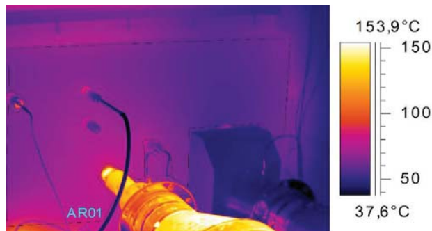
Fig. 8 Combustion Chamber – Right (Air Preheater) Side
