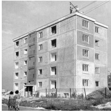
Fig. 1 First ‘panel’ building in Hungary [14]
