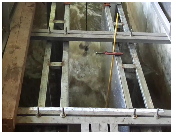
Fig. 6 Turbine placed at the tunnel end
