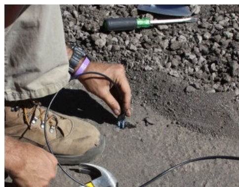
Fig. 3 Installation of a moisture probe
