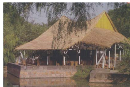
Fig. 7 The bamboo roofs of the Helou Pavilion [10]
