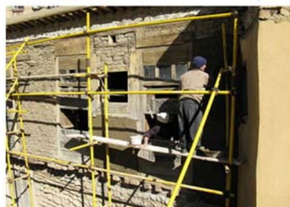
Fig. 9 Ingredients of wall in Masouleh houses
