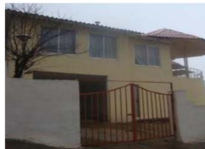
Fig. 14 New construction in staircase structure of Masouleh
