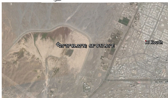
Fig. 1 Google location of the Alkhod Dam in Oman
