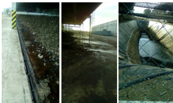
Fig. 1 Leachate generation in waste accumulation areas
