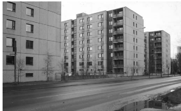
Fig. 1 Typical Finnish concrete apartment buildings from the early 1970's. The buildings have a load bearing bookshelf frame, non-load bearing facades of concrete sandwich elements and self-load bearing balconies
