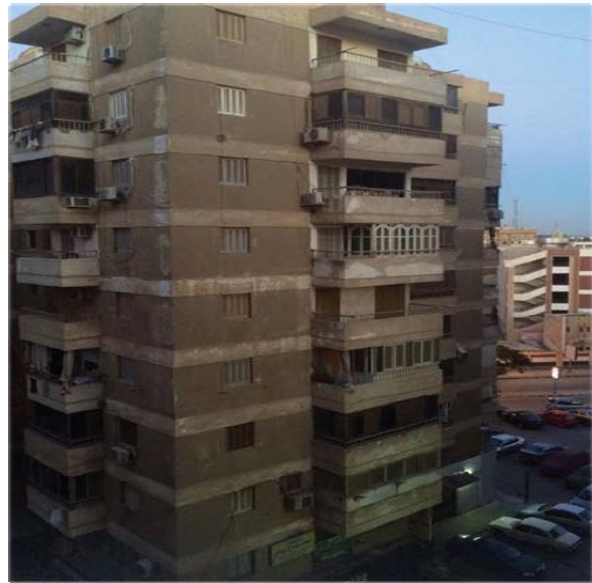
Fig. 5 Changes to a residential building for middle-class residents in Minia City
