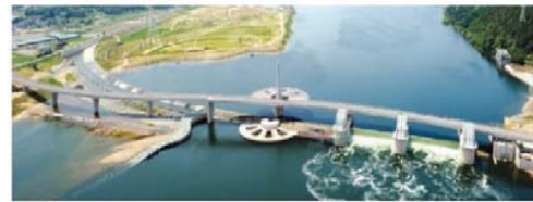
Fig. 1 The focused weir structure
