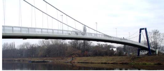
Fig. 9 Three span suspended pedestrian bridge with 159 m deck
