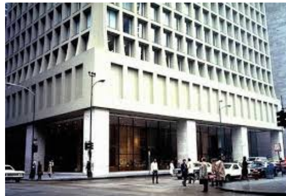
Fig. 2 Continuous deep beams supported on concrete columns
