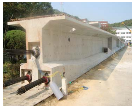
Fig. 12 Field test of anchor head load cell
