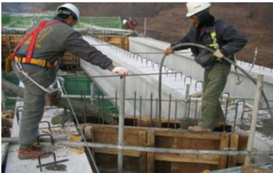
Fig. 2 Placing Diaphragm in Field
