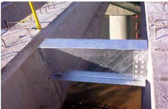
Fig. 3 Steel Cross Beam
