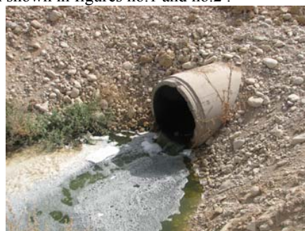
Fig. 1. Effluent of yasuj waste water treatment plant
