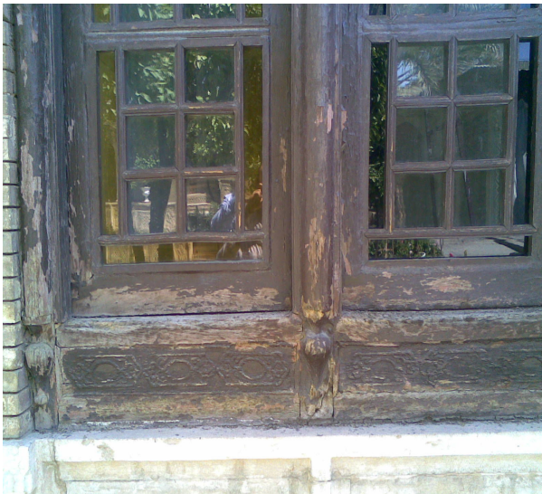
Fig. 5 Decomposition of Wooden door – Ghavam House -Shiraz Esfahan
