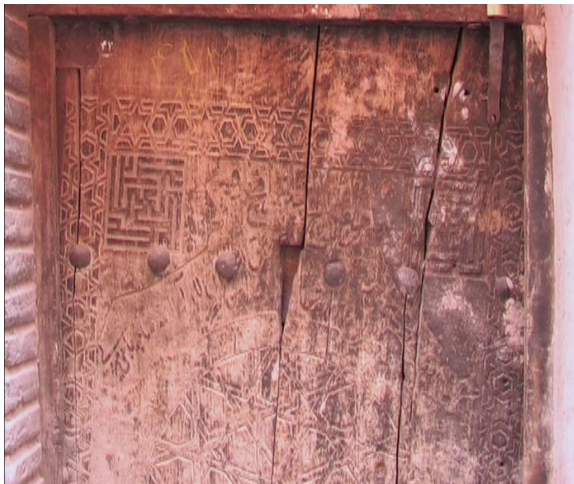
Fig. 2 Decomposition of Wooden door – Abyaneh Esfahan
