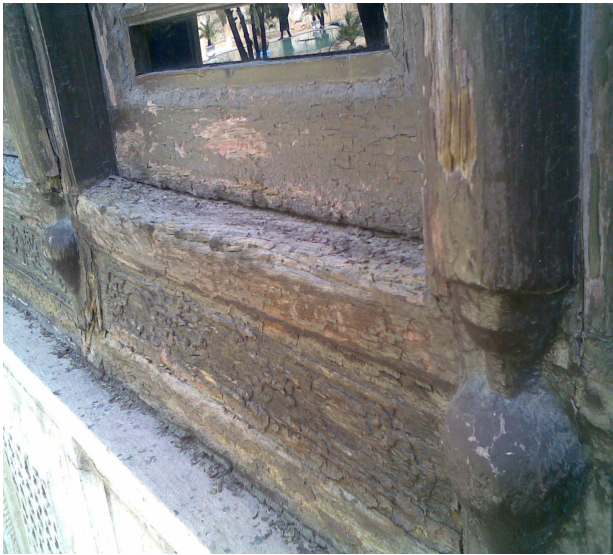
Fig. 4 Decomposition of Wooden door – Ghavam House -Shiraz Esfahan
