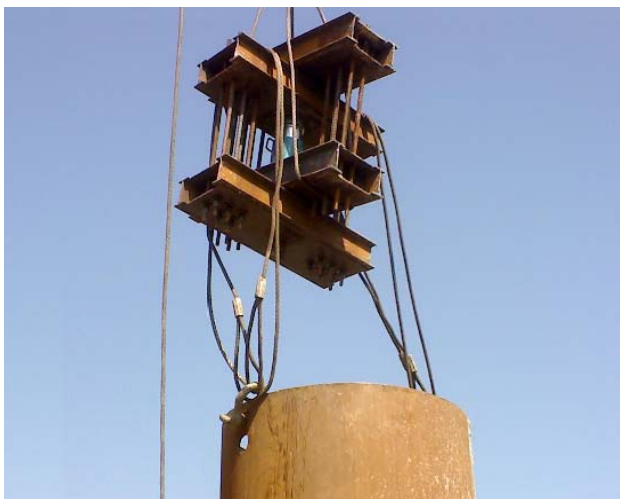
Fig. 3 Imposing tension force to pile
