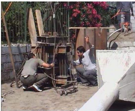
Fig. 2 Hydraulic Jack installation in the frame.
