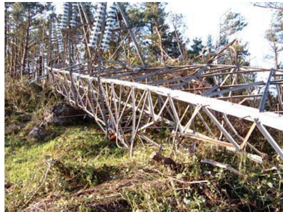
Fig. 1 The collapse of transmission tower by the typhoon 'MAEMI'
