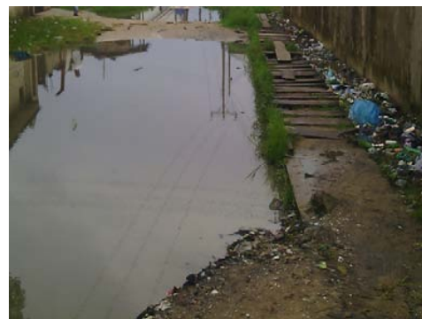
Fig. 1 Abrupt truncation of drainage, that resulted in flooding
