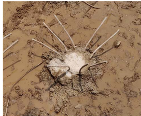
Fig. 2 Condition of prepared pile head
