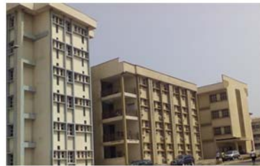
Fig. 3 Egg-crate fins used on building walls in the study area
