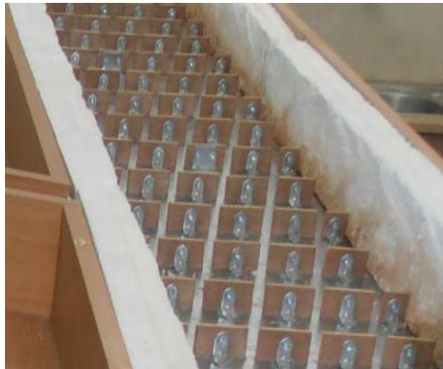
Fig. 3 Photograph of installed baffles (Taken from downstream perspective)
